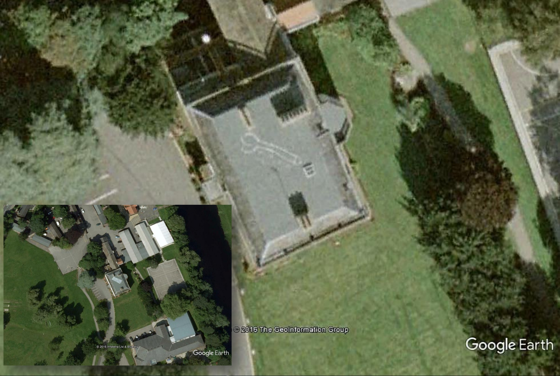
Yarm School roof, Stockton-on-Tees, in 2006, and 2016
